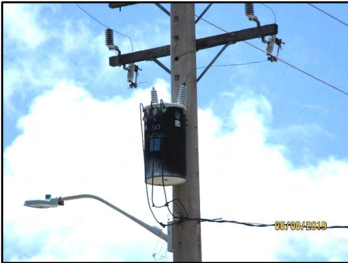
Photograph 17. One pole-mounted transformer was observed to the northeast of the subject property, along University Avenue. Black staining was visible on the exterior of the transformer (09 May 2019).
