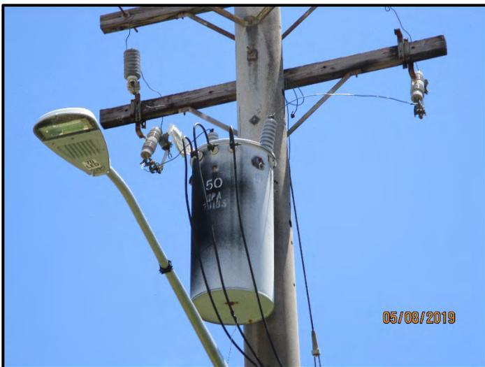
Photograph 18. One pole-mounted transformer was observed to the south of the subject property, along Atbut Lane and at an apartment building. Black staining was visible on the exterior of the transformer (09 May 2019).
